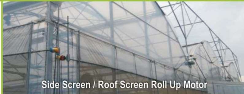
SIDE SCREEN / ROOF ROLL UP AUTOMATION
